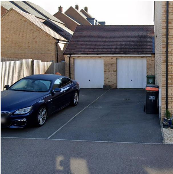
Properties designed with limited frontages and no rear access result in wheelie bins stored in driveways, and vehicles parked on-street.
