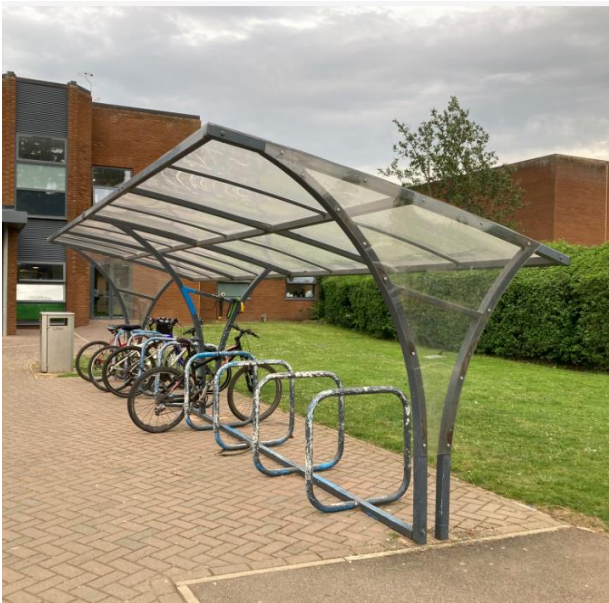
Sheffield stands under a shelter at a leisure centre provide good short-term parking for visitors, located close to the main entrance.
