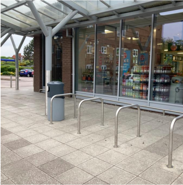
Short-term cycle parking located outside a supermarket. The cycle parking is under a canopy, is closer to the main entrance than any car parking spaces and is located so as not to block access for pedestrians.
