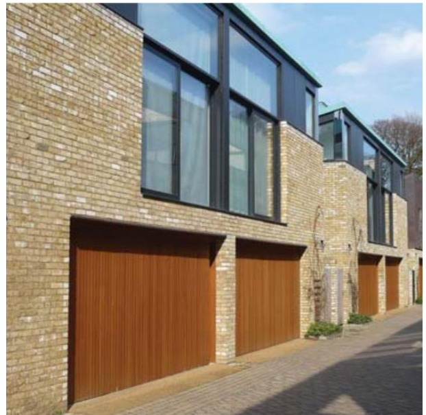
Wide garage doors allow access for a car and cycle independently of one another.
