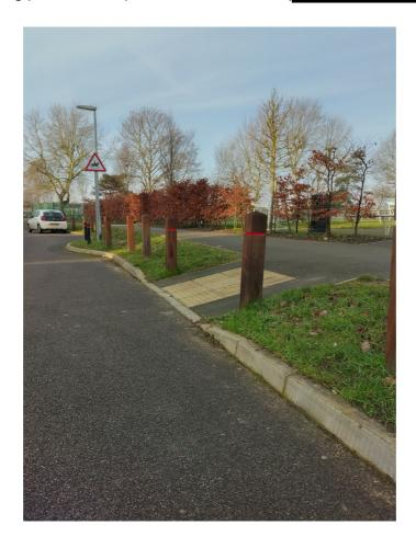
10) Connecting footpath from (King's Reach): no dropped kerb for pedestrians at end (also inconvenient for workers who surfaced it, they had to move a heavy roller from the nearest dropped kerb, causing minor damage to the surface - white marks); also has only been surfaced to footpath to short section to is still unsurfaced.
