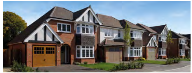
Detached block: in lower density areas blocks can be defined with detached homes. Here parking is provided in a convenient and practical location close to the front door between landscaped gardens.
