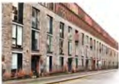
1. Perimeter block: A strip of development around a private courtyard/gardens. The private interior is not accessible to people from outside the scheme. It includes private and communal gardens and car parking.
